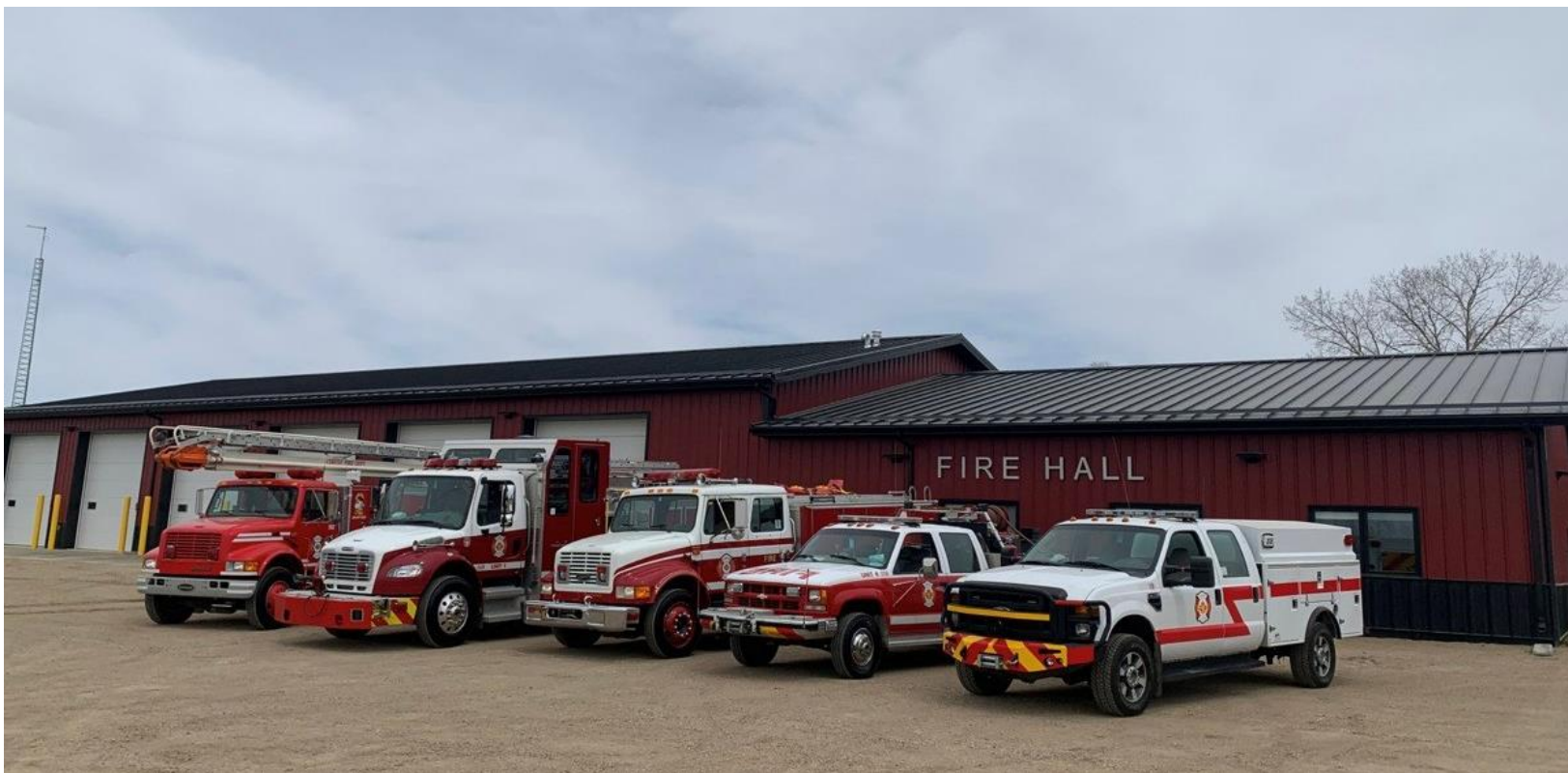
The new Fire Hall is three times the size of previous facility to better serve Carlyle and the surrounding region.
